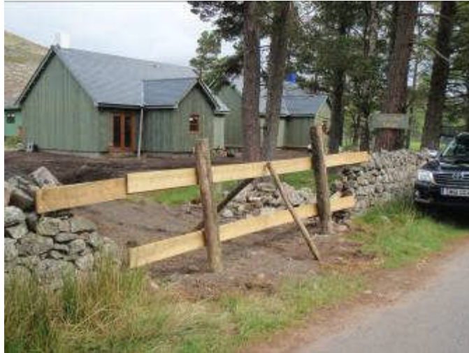
Fig. 3 : currently blocked opening in drystone wall
